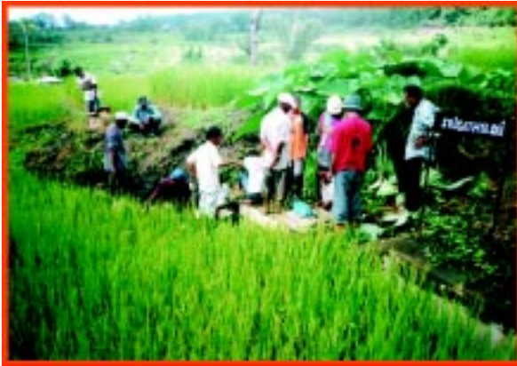
Work in progress for providing water to a remote area in Indonesia.
