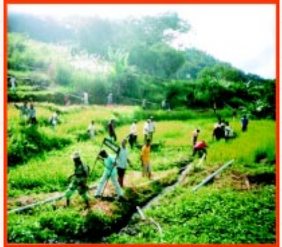
Laying of pipes being undertaken by Sri Sathya Sai Organisation of Indonesia.
