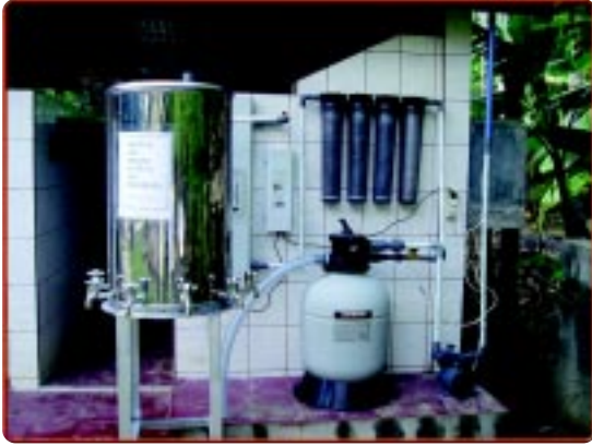
Water purification unit installed by the Medan task force in North Aceh.
