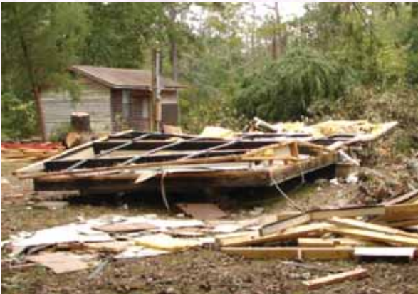
A scene of devastation caused by Hurricane Katrina in the U.S.A.
