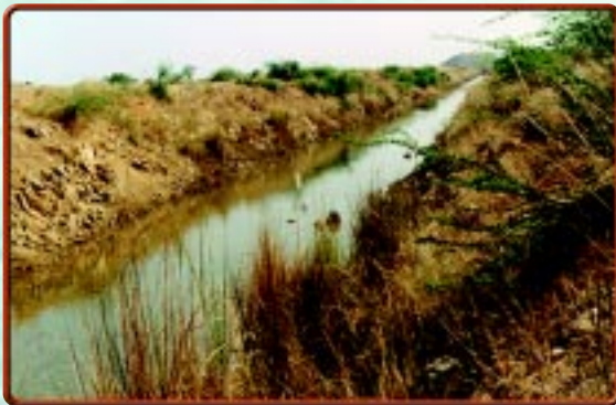
Part of Kandaleru-Poondi Canal before concrete lining.
