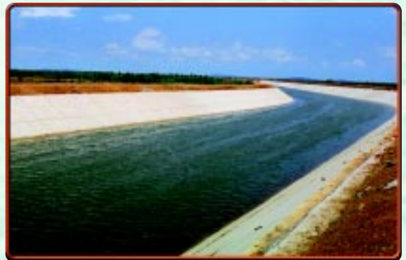
The Canal (now christened Sri Sathya Sai Ganga Canal) after concrete lining.
