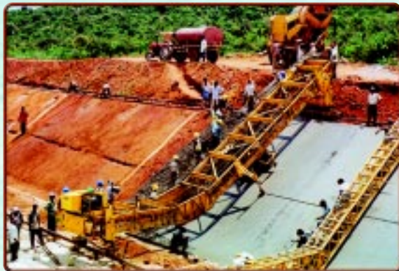
Concrete lining of Sri Sathya Sai Ganga Canal was a huge task.
