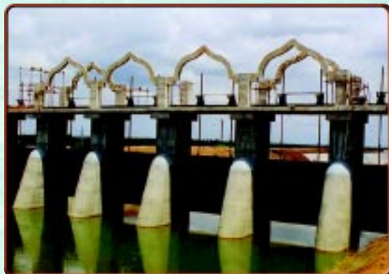
An Escape Regulator constructed on Sri Sathya Sai Ganga Canal.
