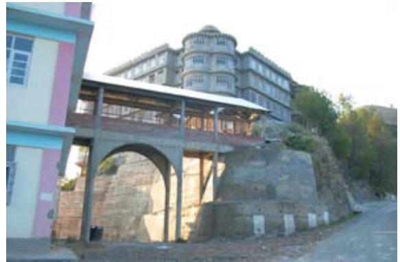
The interlinking corridor which links the school and the hostel. The hostel building is seen in the background.
