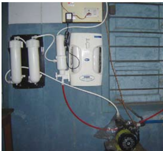
Nine villages were provided pure drinking water by the Sai Organisation of Tamil Nadu by installing water purification plants in them. The picture shows a water filter installed in a village school.
