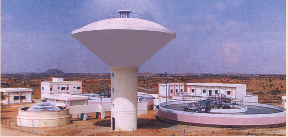
Water Treatment Plant at PABR for Anantapur Water Project.
