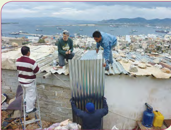
Sai devotees repaired the home of a needy family in Greece on 2nd April 2011.
